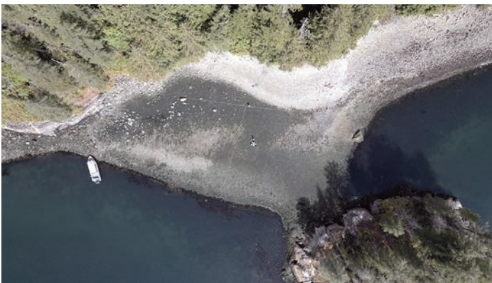
Aerial view of a 2200 m 2 Loxiwe at low tide in Phillips Arm, British Columbia. The outer perimeter of this Loxiwe is a rock wall, at the water's edge, constructed thousands of years ago by the people of this area. The rock wall serves to flatten and extend the beach by catching sediment at the ideal tidal zone for clam habitat (i.e., 0.7-1.5 m above sea level).
